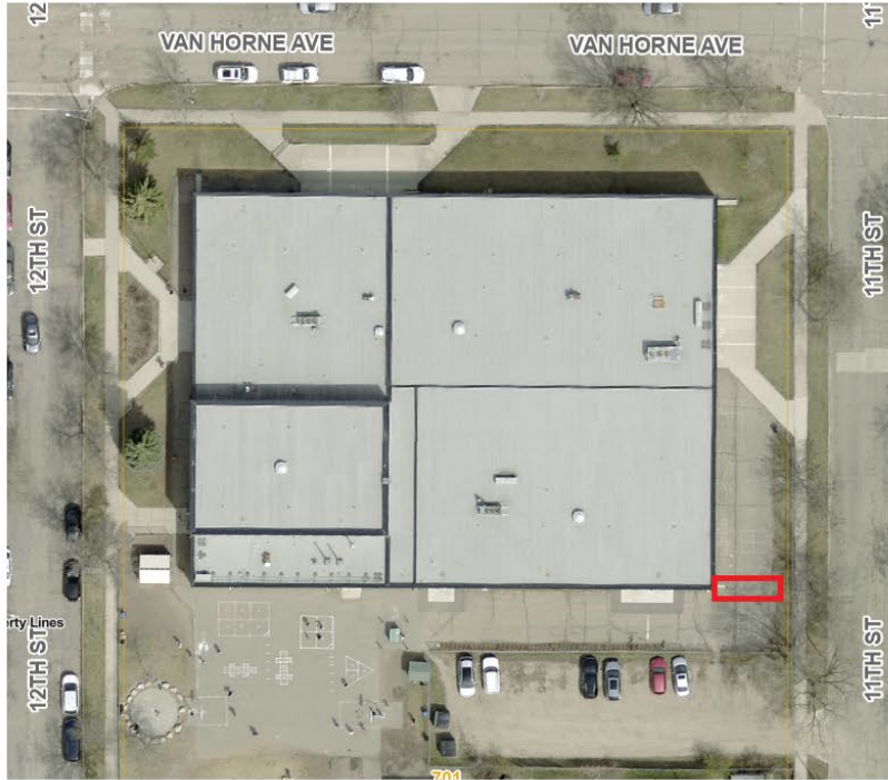
Betty Gibson School Drainage Grating
